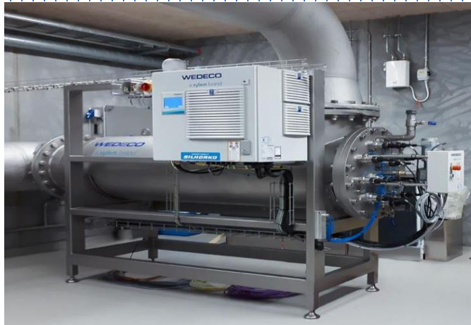
Ultraviolet water disinfection system
