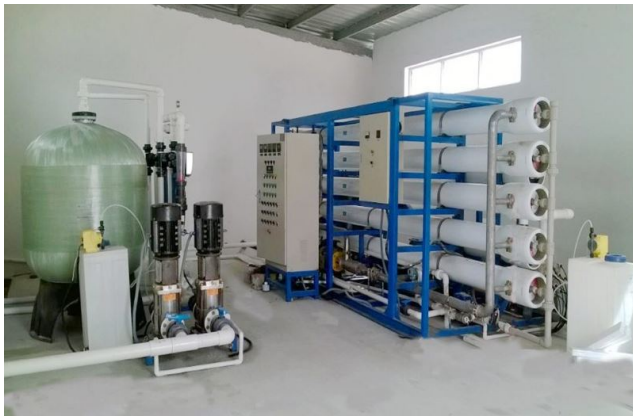
Pic.2 Reverse Osmosis Cleaning Equipment
